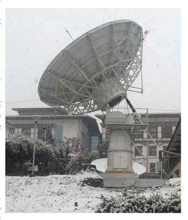
The reflector panels are stretch formed to give surface accuracies below 0.3mm RMS, antenna efficiency better than 60%. 16 nos of high strength doubly curved aluminium stretch formed panels on 16 nos radial trusses emanating from a center hub constitutes the reflector. The hub can house Receive/ Transmit electronics.
